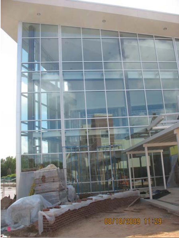
Curtain-wall ASTM intrusion testing
