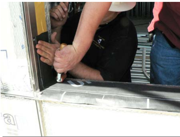
Field Training of installation critical trades
