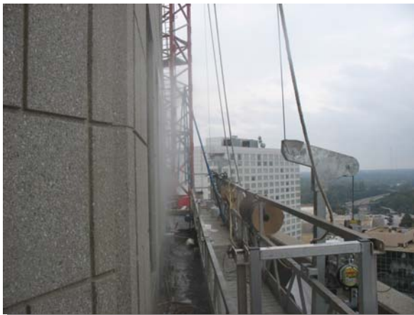
42 Storey The Mansion ASTM E1105 Test Atlanta, GA
