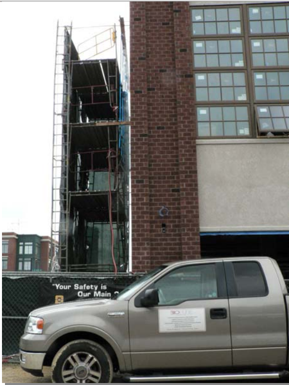
Full-scale façade water intrusion test Charlotte, NC
