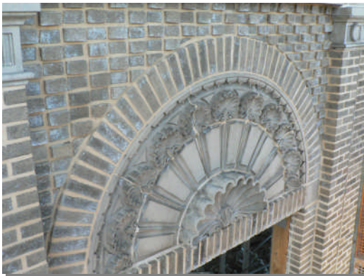
Masonry clay units and limestone restoration.
