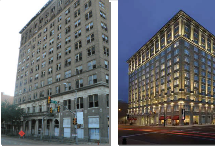
Before and after, preservation of the historic façade.
