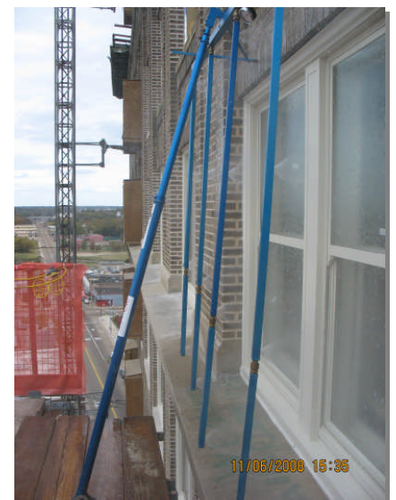
Water intrusion testing of the façade.
